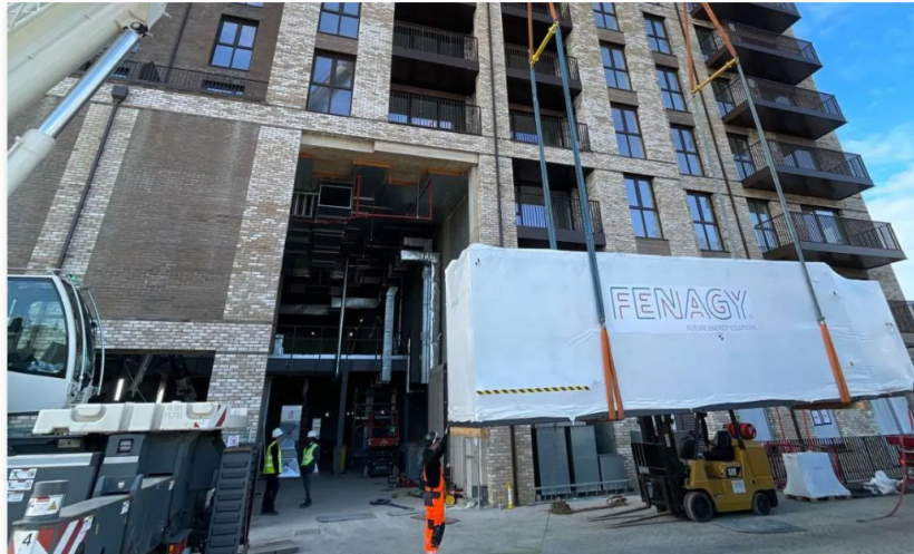
A Fenagy CO 2 heat pump being installed in Clapham Park. Photo credit: Hemiko
